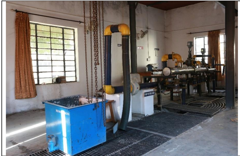
Fig3: Pump Testing Lab
