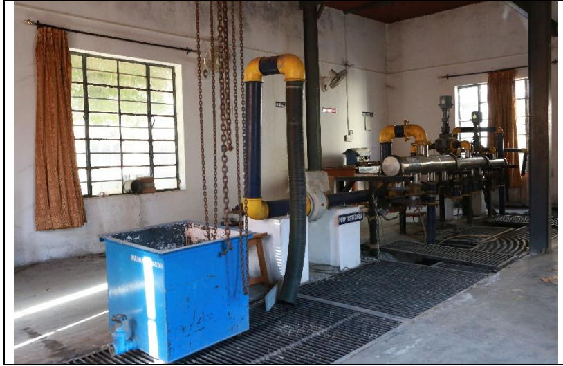
Fig 4: Pump Testing Lab
